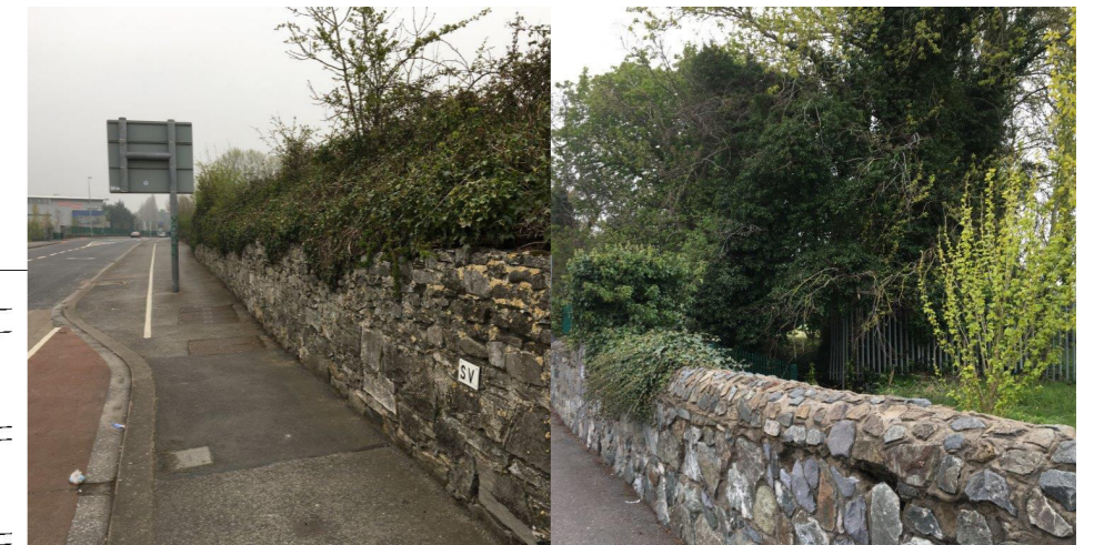
Existing stone wall along eastern boundary
