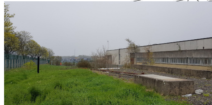
Existing factory building
